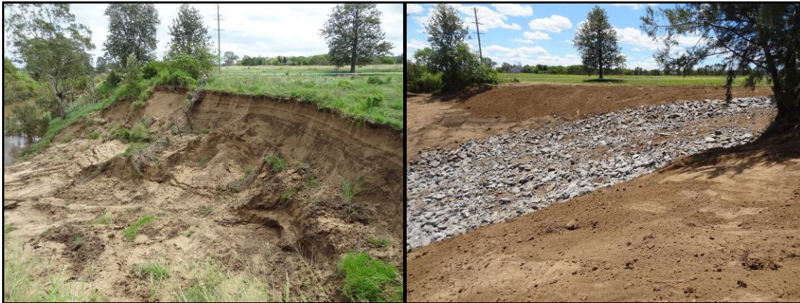
Figure 4: The larger Reach affected by fluvial scour – (a) prior to restoration; and (b) nearing completion of restoration earthworks
